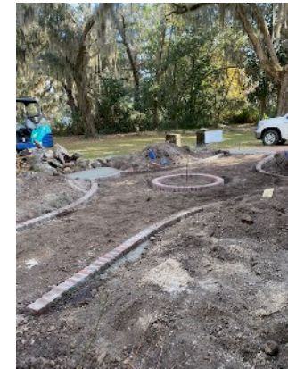
Walkway's brick edging going in.
