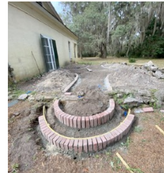
New steps being outlined and tied into the front walkway.
